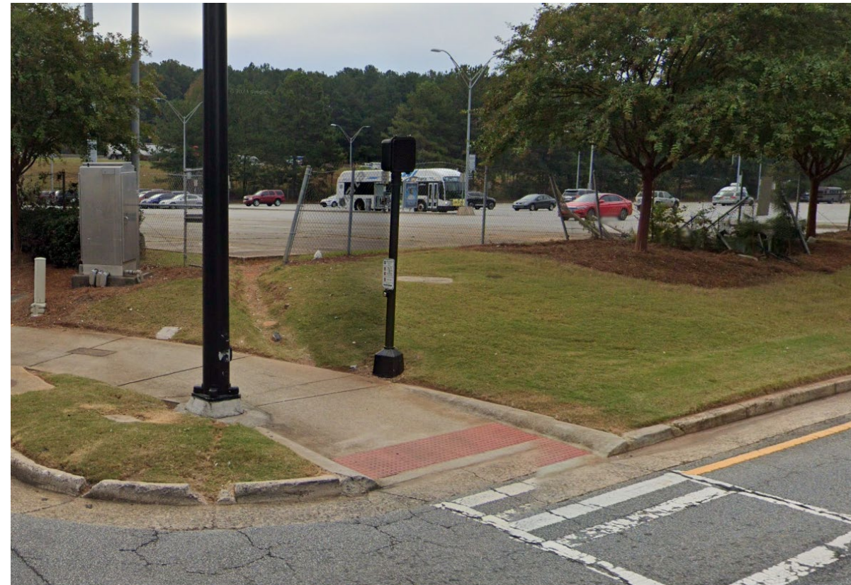
Pedestrian access needed for heavy foot traffic at NW corner of Mansell Road Park and Ride
