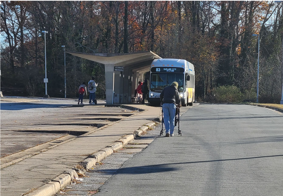
Deteriorating sidewalk and missing ADA Ramps at Barge Road Park and Ride
